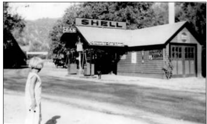
Gas Station in the 1930s
